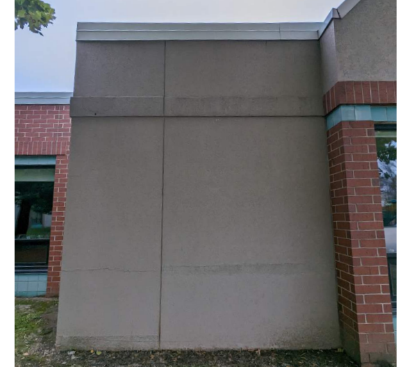
DEGRADING AT GROUND
