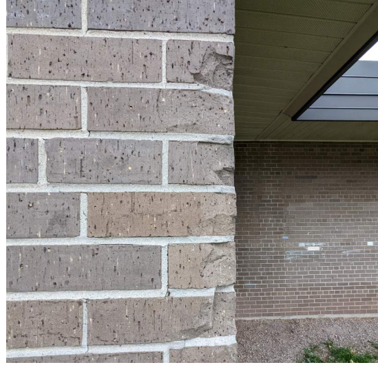
CHIPPING AND TUCKPOINTING
