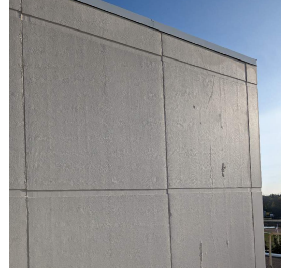
CRACKS (NON-STRUCTURAL)
